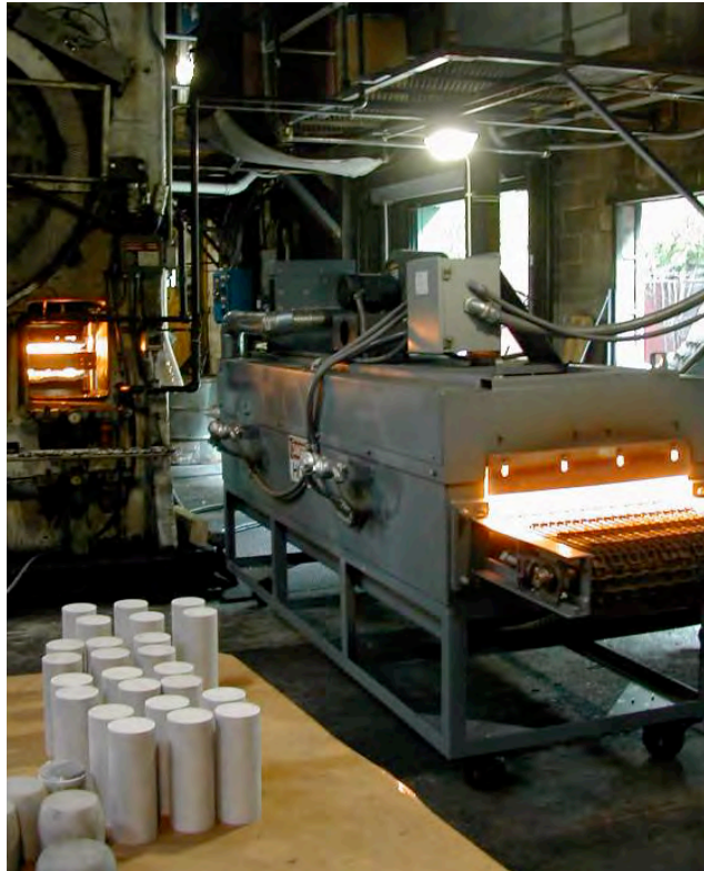
Figure 6.I.8 Continuous-belt IR heating furnace installed at Queen City Forging Company, Cincinnati, Ohio. 93
